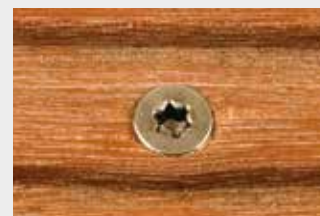
Pilot-drilling + Terrassotec screw
