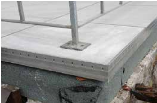
Example of application aluminium eaves
