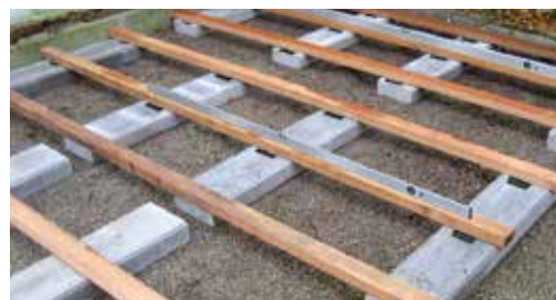
Rolfi spacer in combination with timber substructure.
