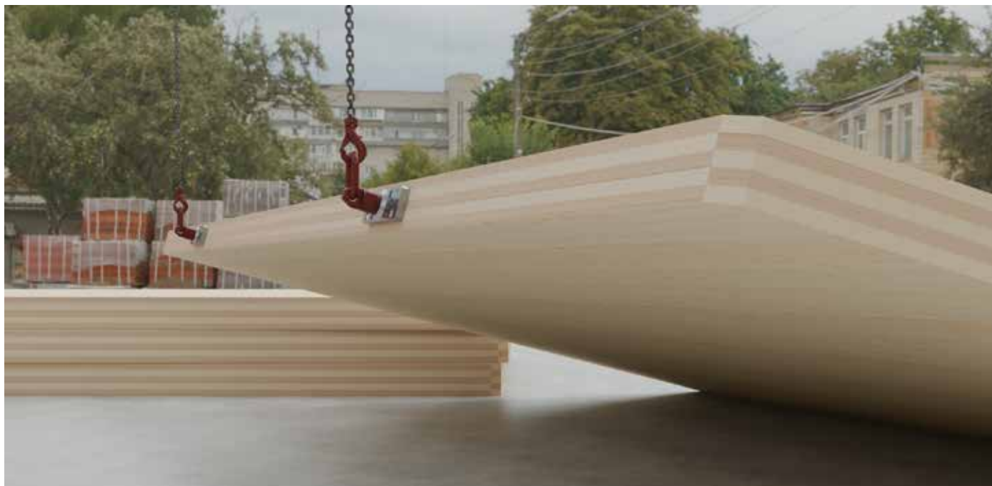
Powerblock transport anchor in use.
