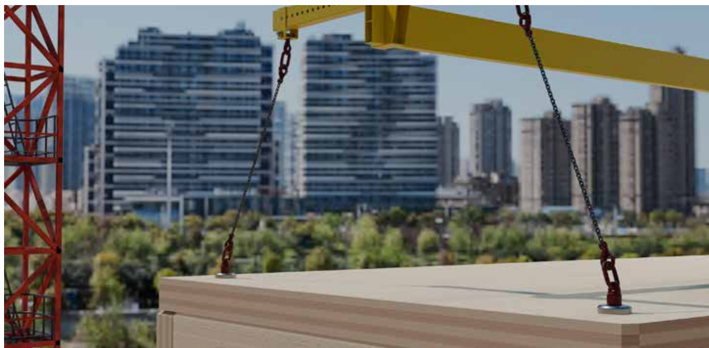
Powerring transport anchor in use.
