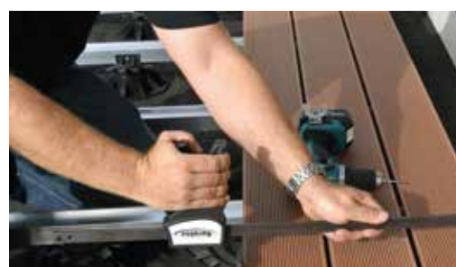
Example of application tension clamp
