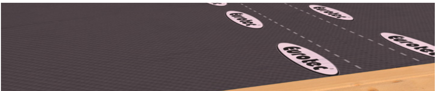
Formwork and foil on the existing ceiling
