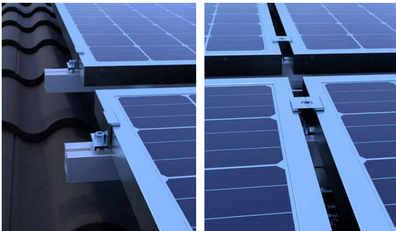
Eurotec end/centre clamp installed on the installation profile, to fasten the solar modules
