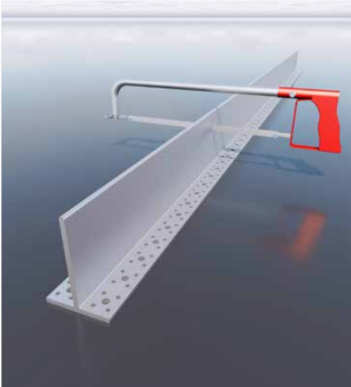
Individual cutting of the profile to length
