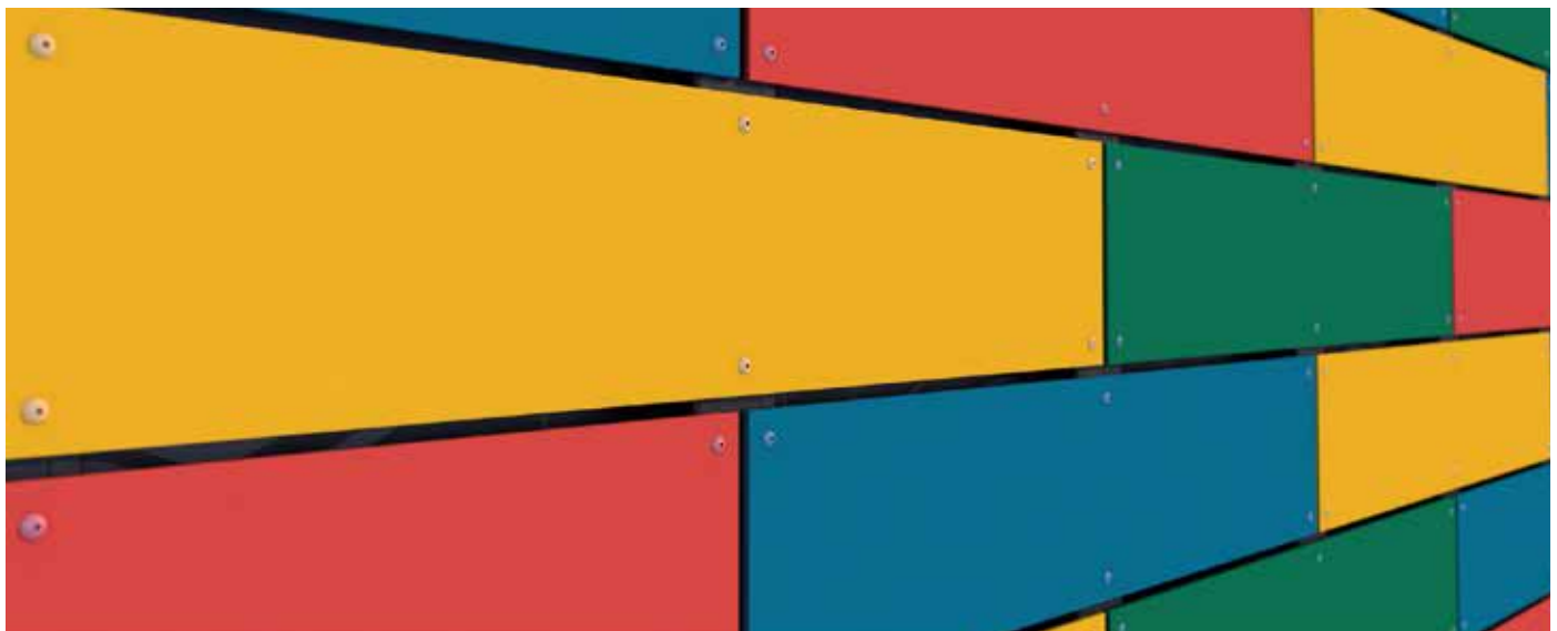
High-pressure laminate (HPL) panels fastened with coloured façade screws in the appropriate colours.
