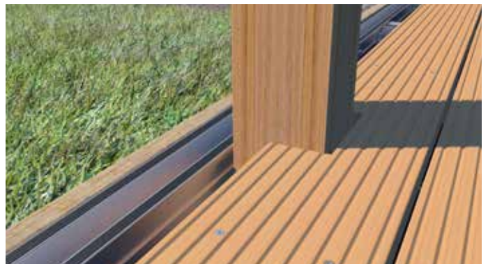
13 Saw notches for posts.
