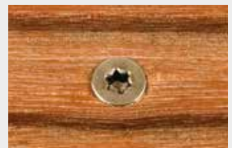
Pilot-drilling + Terrassotec screw
