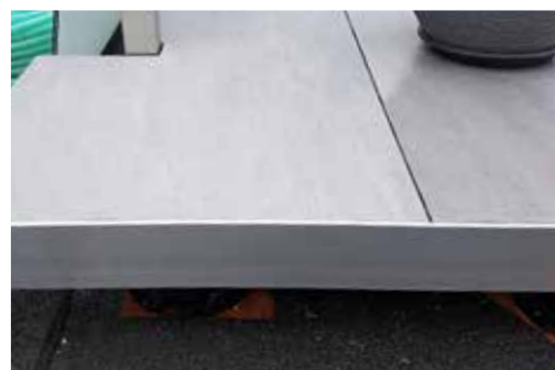
Example of application aluminium cover
