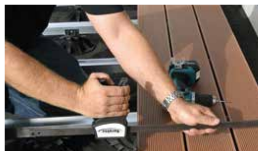
Example of application tension clamp
