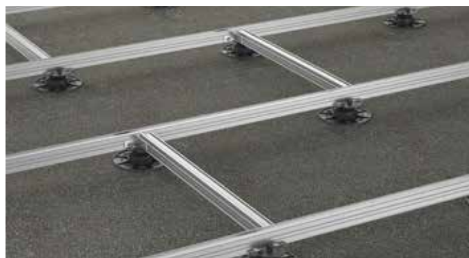
Adjustable pedestal BASE with aluminium system profile EVO Light
