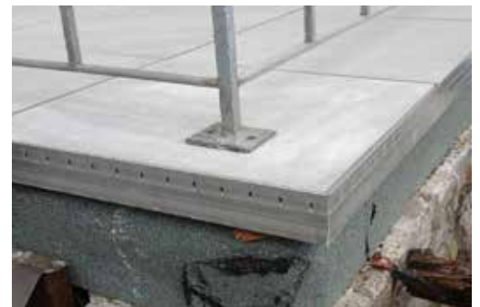
Example of application aluminium eaves
