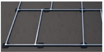
**STEP 1:** Connect the laid-out mounting profiles using corner and T-connectors. In addition, place a load distribution plate under each of the connection points.
