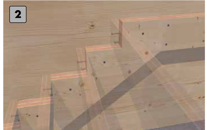
Attach the step end cap to the front of the step support.
